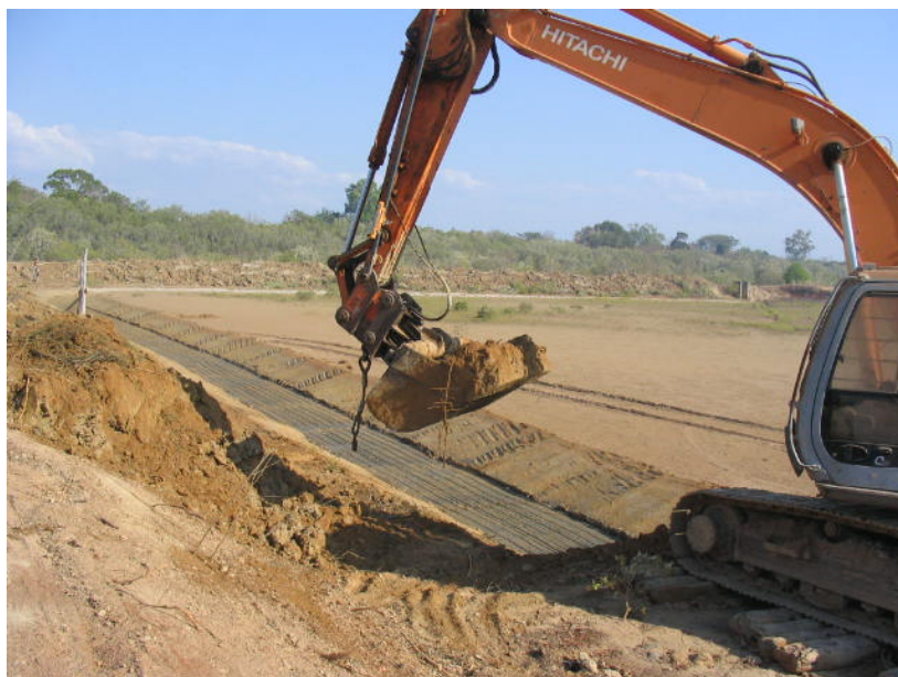
Figure 10 Draining moat excavated around the internal periphery of production ponds. (Source : Gwalwa Daraniki Enterprise Pty Ltd , Mudla farms Mud crab Project, Progress Report 1, December 2005)
